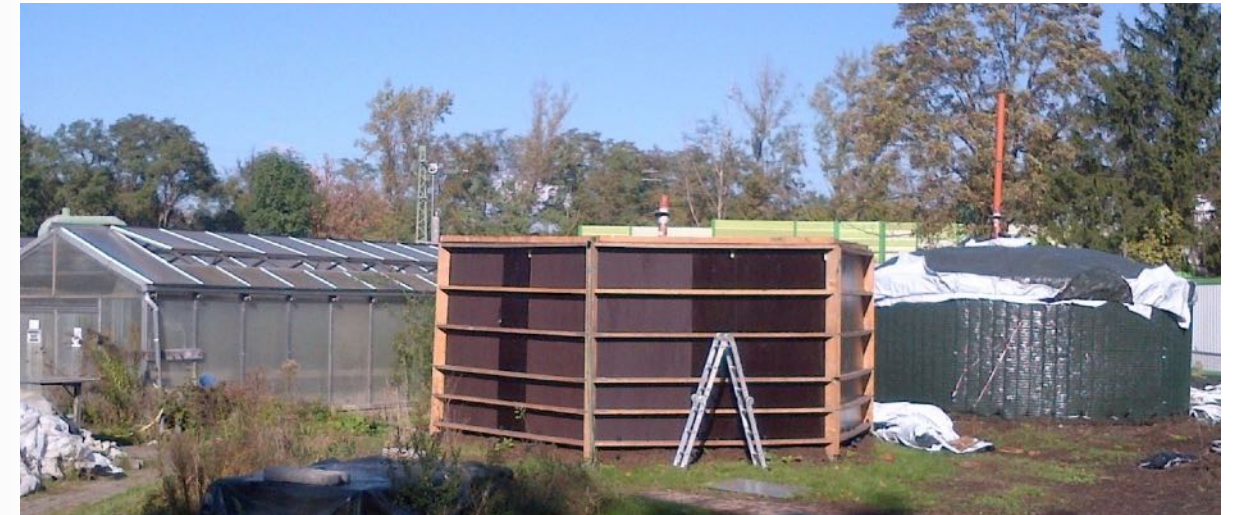
Figure 2. Construction of a prototype with modular wall elements in wood construction (still without panelling). In the background: The three-aisled greenhouse to be heated and a round Compost heater made of double-bar fence elements with horizontal heat exchanger.
